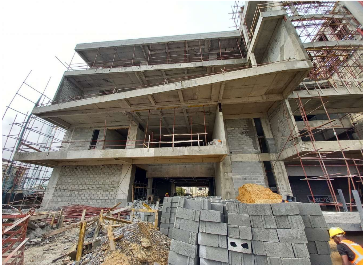
3-6m cantilevers at building Approach -Left
