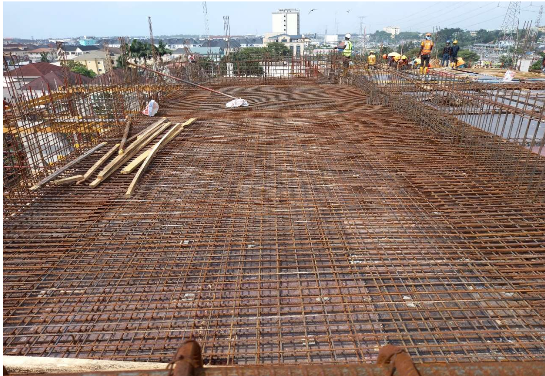
Reinforcement Arrangement in the Suspended Swimming Pool
