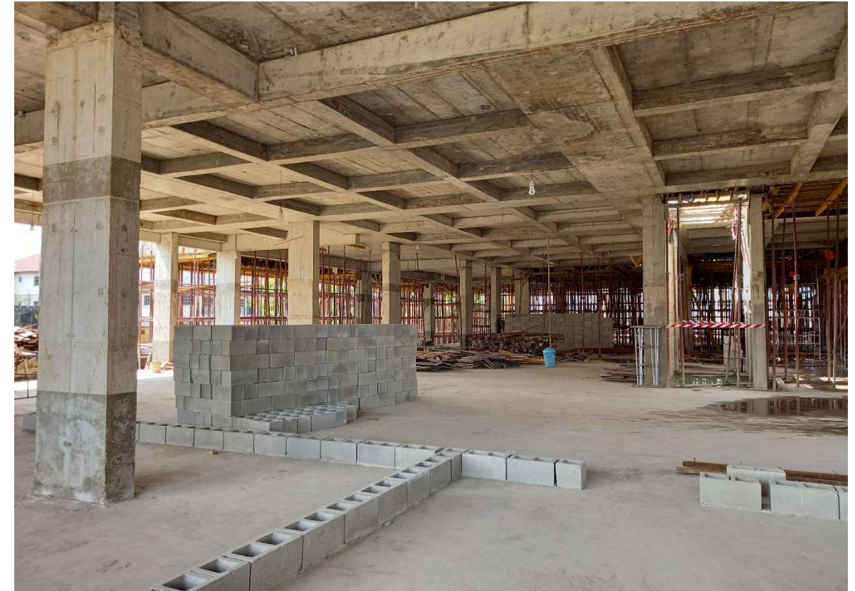
1 st floor level soffit after removal of forms and props
