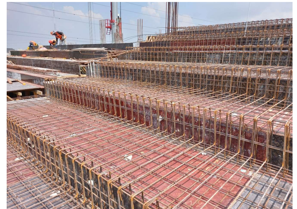
Reinforcement Arrangement of Cinema Gallery
