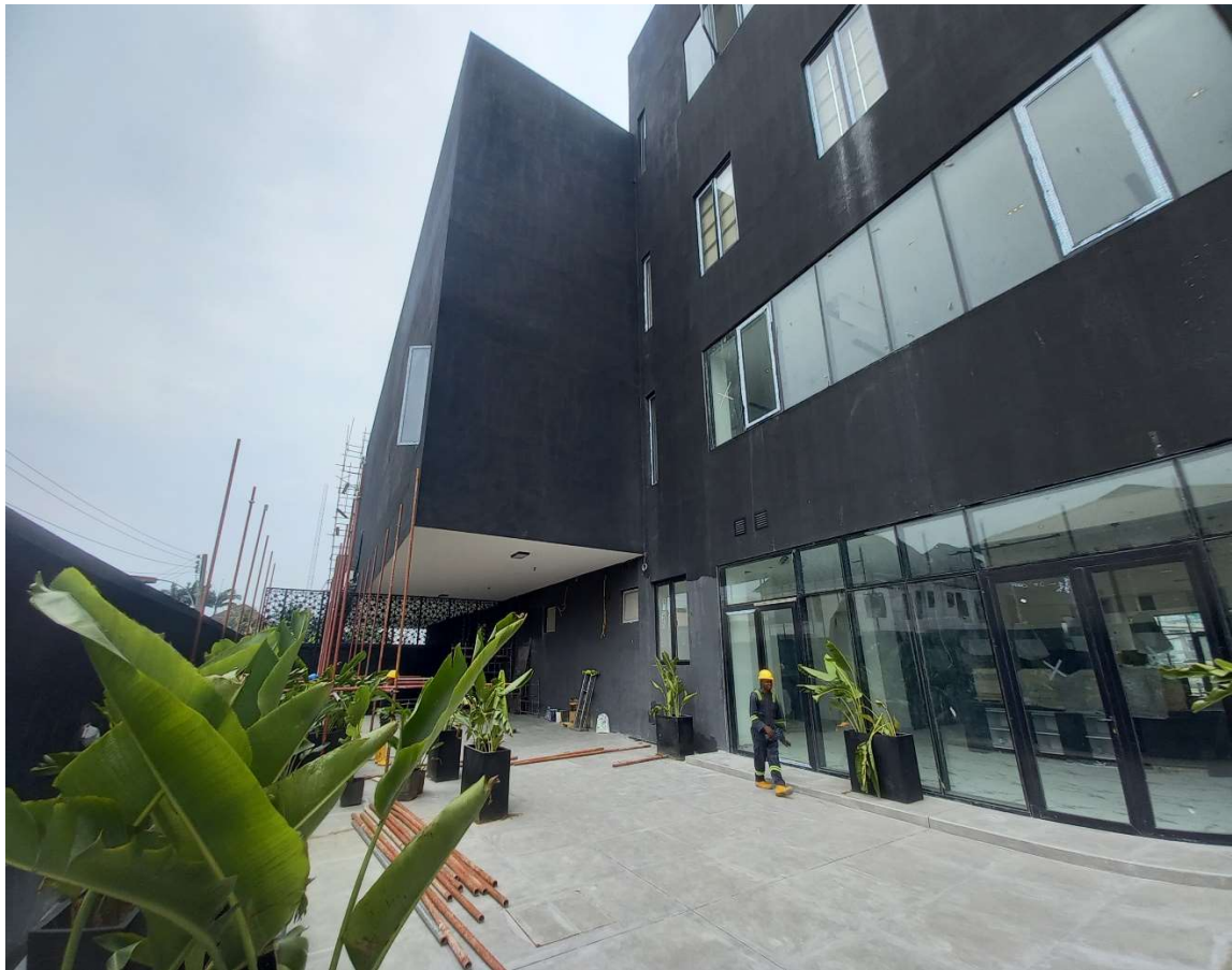
6m Cantilevered Building Rear
