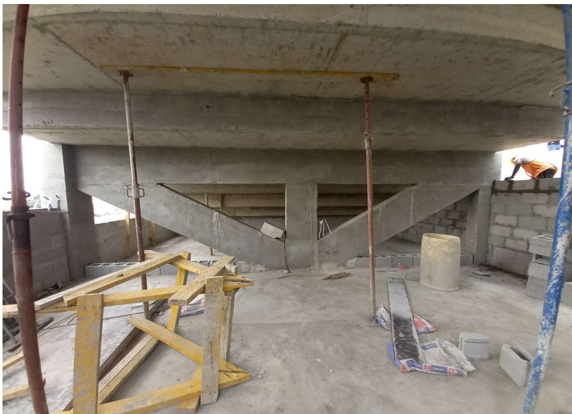
Concrete Truss System Beneath Cinema Gallery
