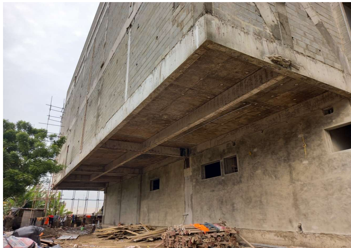
6m Cantilever at building rear
