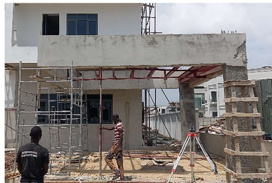
Figure 4: Car port after de-propping
